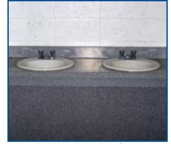
West High New Bathroom Sinks
