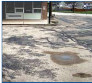
Schneider Playground Before
