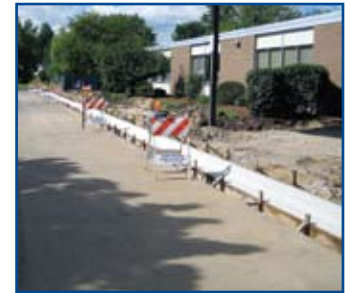
Schneider Pavement Work
